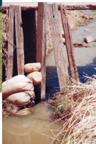
The sluice gate for controlling the flow of water in and out of the Débaré pond (Batamnai village) was badly broken down before the project.
