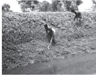
Working on pond banks to ensure the correct slope.
