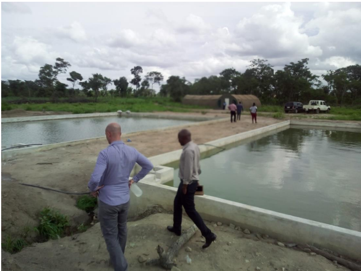
Figure 13 Concrete ponds (30 m X 20 m) constructed for production and practical purposes
