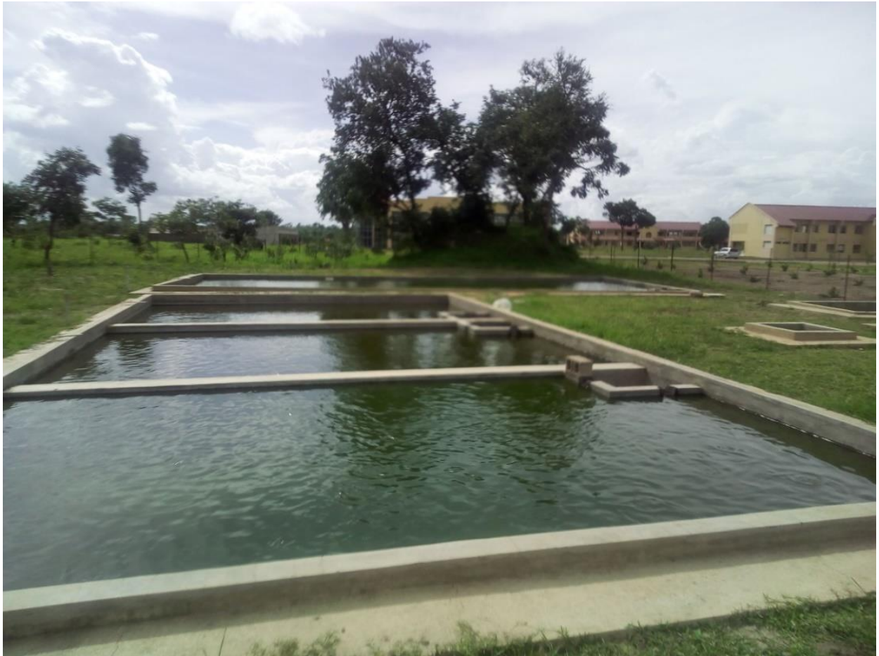
Figure 14 Concrete ponds initially constructed at the front of the institution
