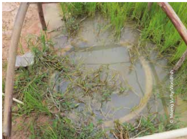
Earth outlet/inlet at Trapaing Thlok Meanchey CFR, Kampong Thom
