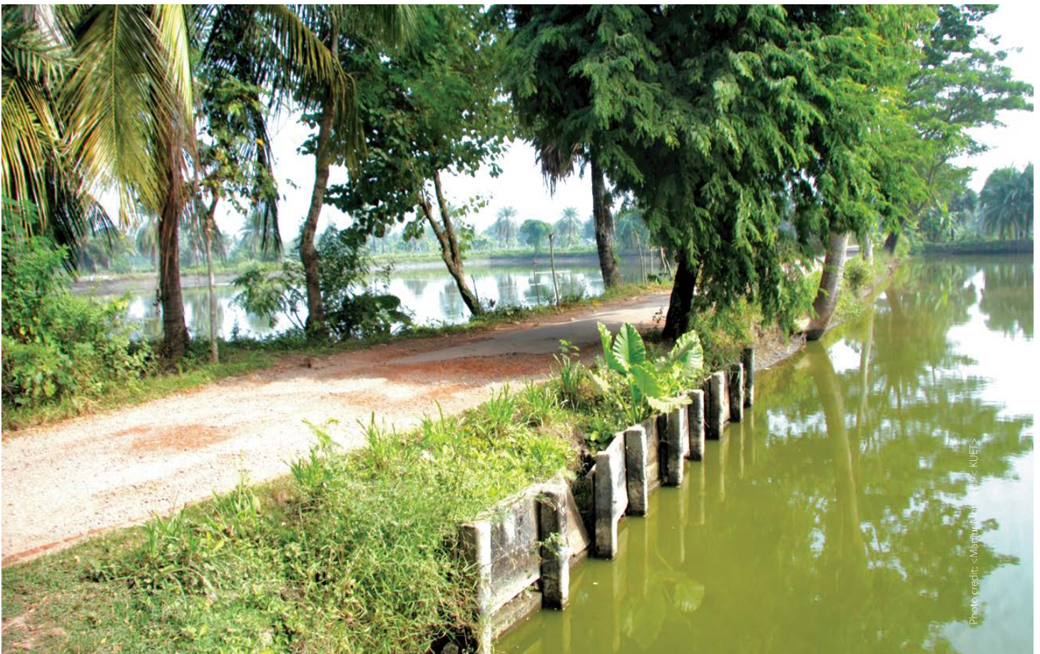
Figure 14. Road blocking cross-flow of water.
