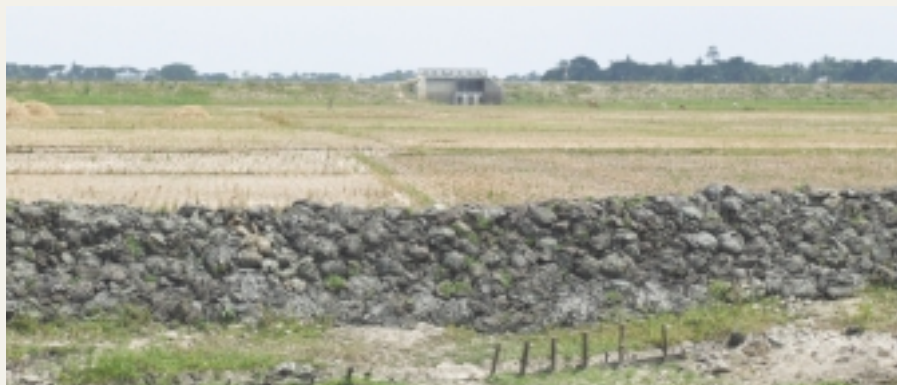
Construction of embankment and sluice gate for floodplain aquaculture
