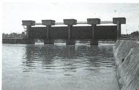
Different faces of Laguna de Bay. Lower photo shows the controversial Napindan Dam, built to prevent entry of saltwater into the lake and render the lakewater suitable for domestic consumption.
