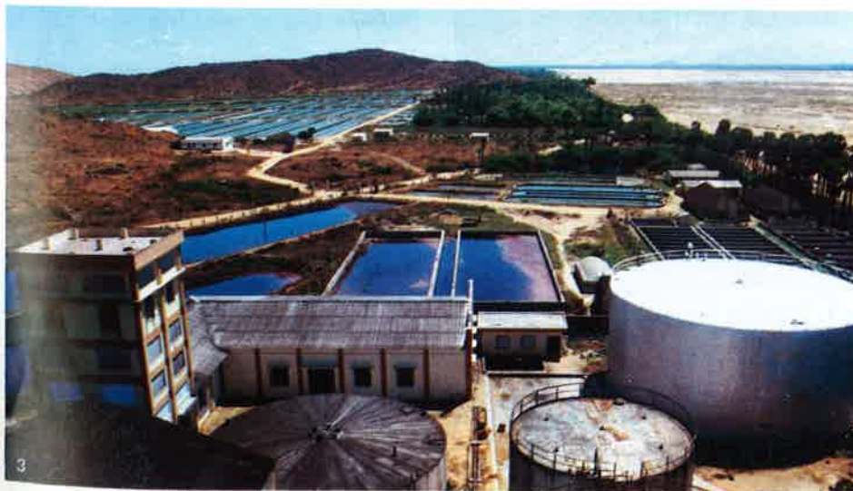
(1) The floating aerator at work. (2) An overview of the fish farm. Note the "bioreef" in the middle of each pond. (3) The VCDL alcohol plant, with the fish farm in the background.
