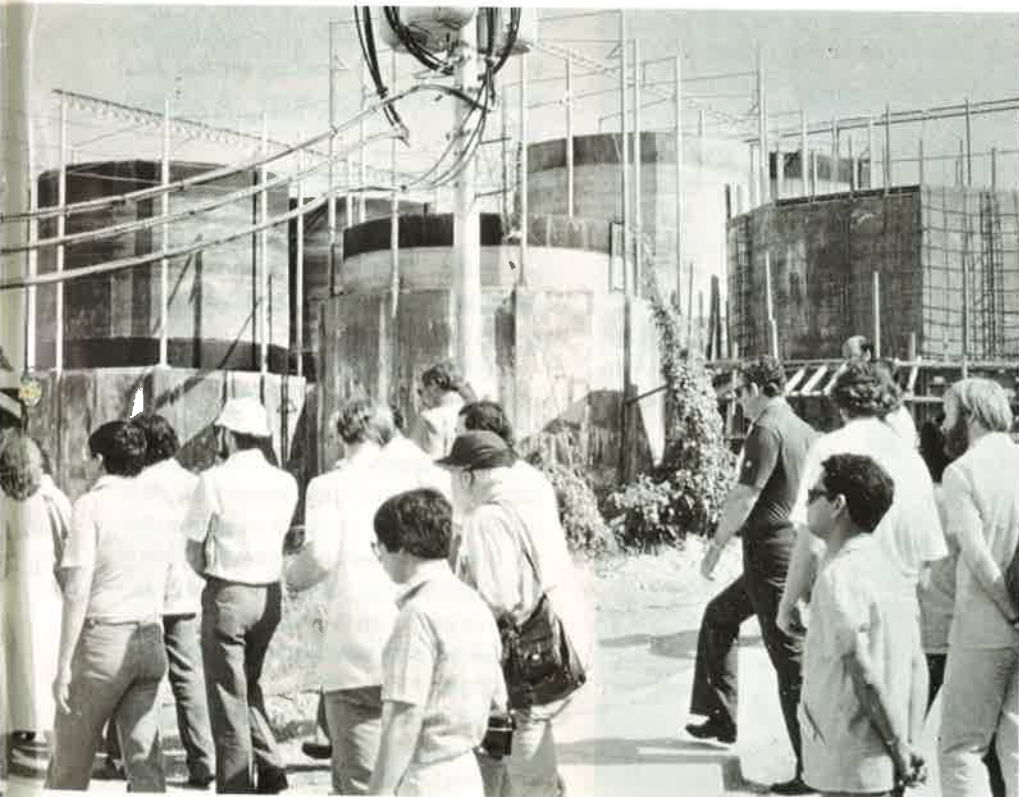
Participants visit Maya Farms, a large piggery complex powered almost exclusively by biogas. Residue from the digesters is also dried and makes up 10% of the pig feed. Photo by I.R. Smith.
