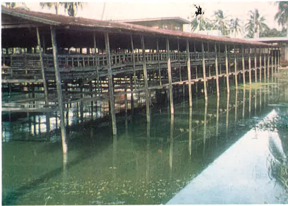
Chicken and Clarias catfish integration in Pathumthani. Chicken coops are constructed above the pond.
